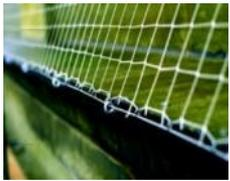
The netting is constructed of a high density polyethylene (HDPE) that is rot proof and UV resistant. It is available in black, stone and translucent (white) and can be flame retardent if necessary. You can expect 10 - 15 years working life from a correctly installed netting system.
