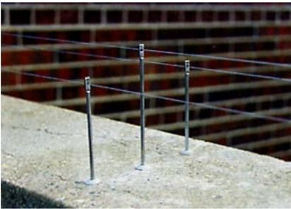
The concept is to place thin stainless steel wires, tensioned with springs, just above the roosting ledge. The wires present an unstable barrier and deter them from roosting.
